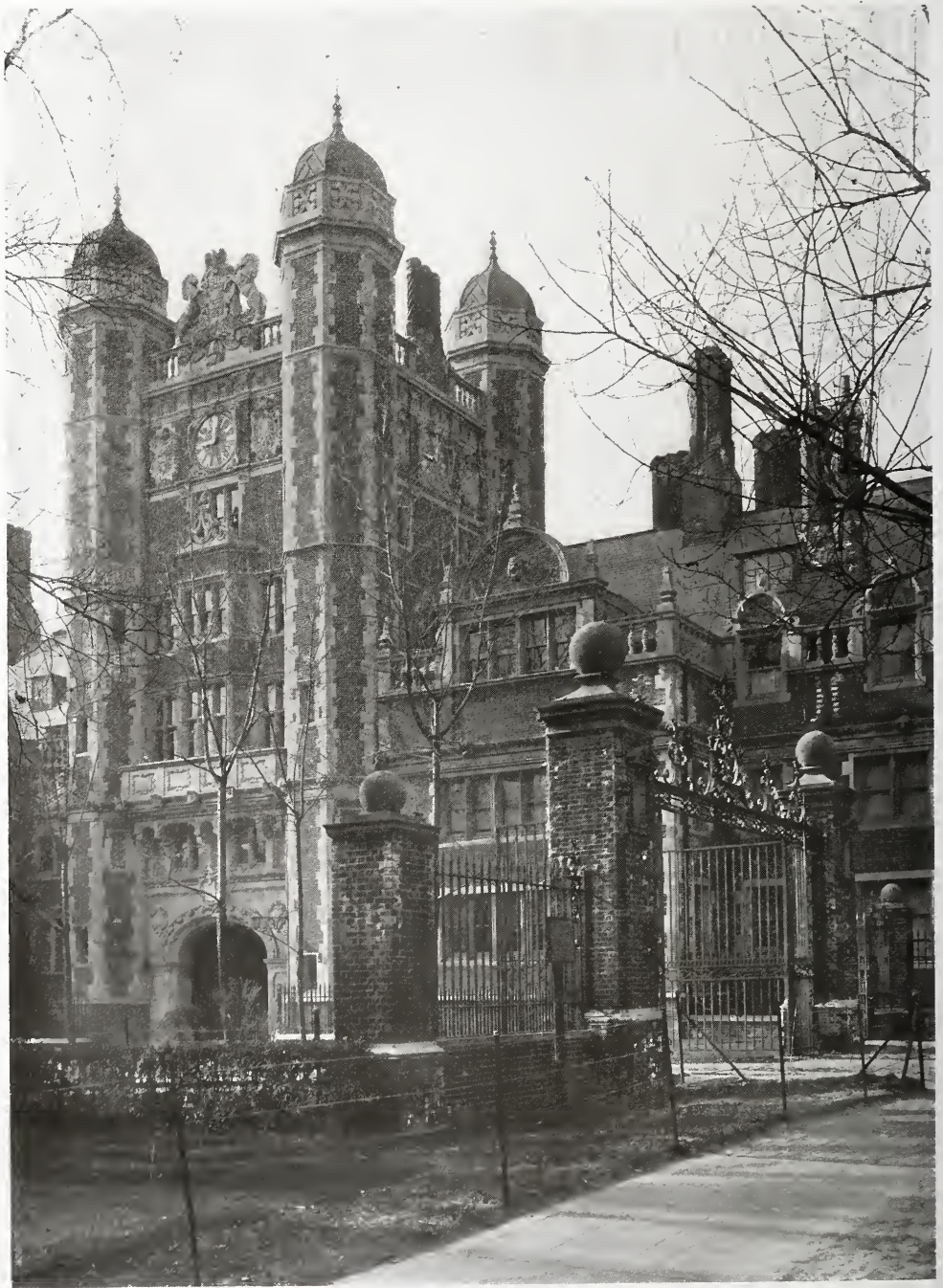
PROVOST'S TOWER—UNIVERSITY OF PENNSYLVANIA. Philadelphia, Pa. Cope & Stewardson, Architects.
